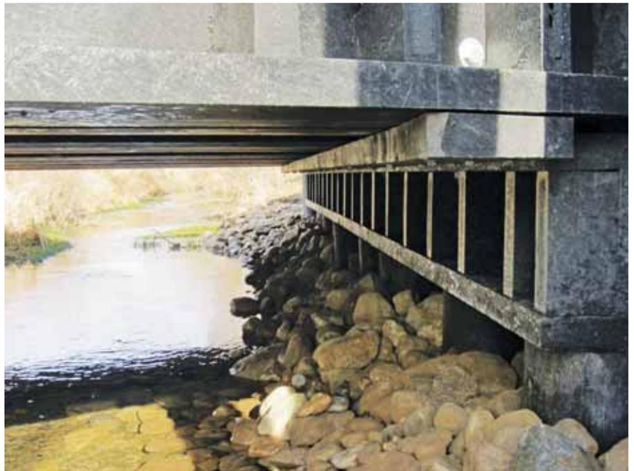
the Onion Ditch Bridge is all plastic, abutments to guardrail.
