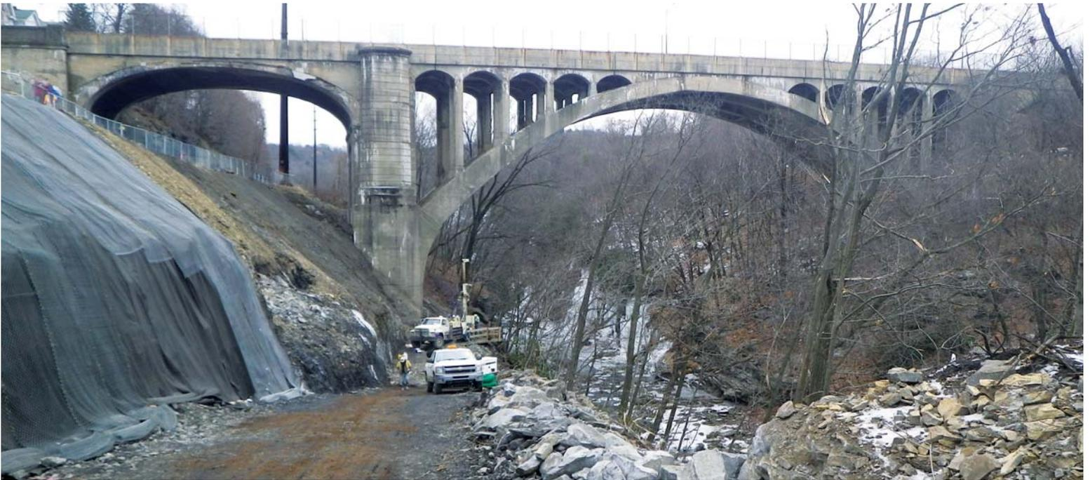
**A condition survey concluded that the upper portions of the bridge, including the deck beams, deck arches and deck itself required complete replacement.**
